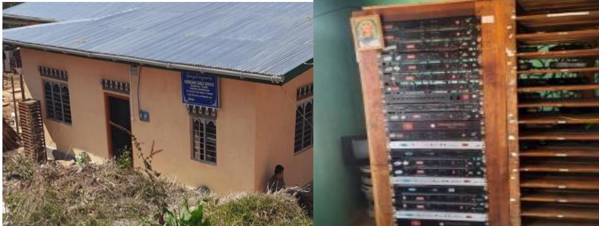
Figure 4. New Office of Kuenzang Cable Service Figure 5. Control Room of Kuenzang Cable Service
