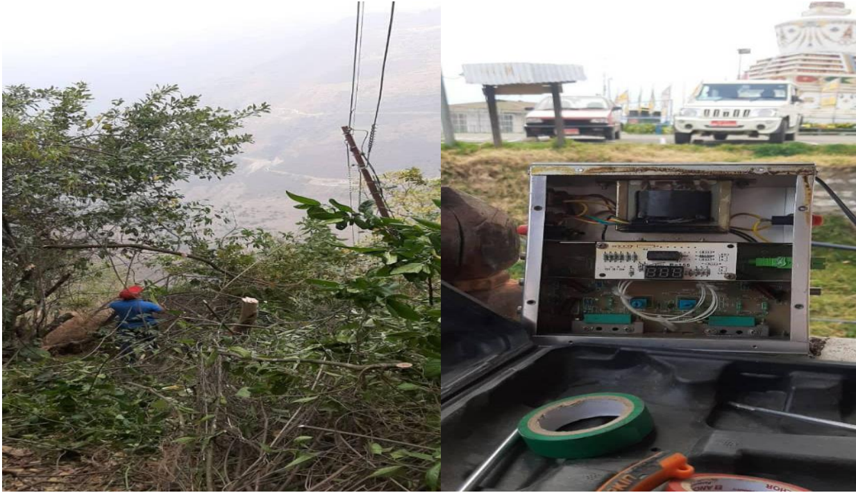
Figure 9. LCOs doing the cable maintenance (23 March, 2022)
