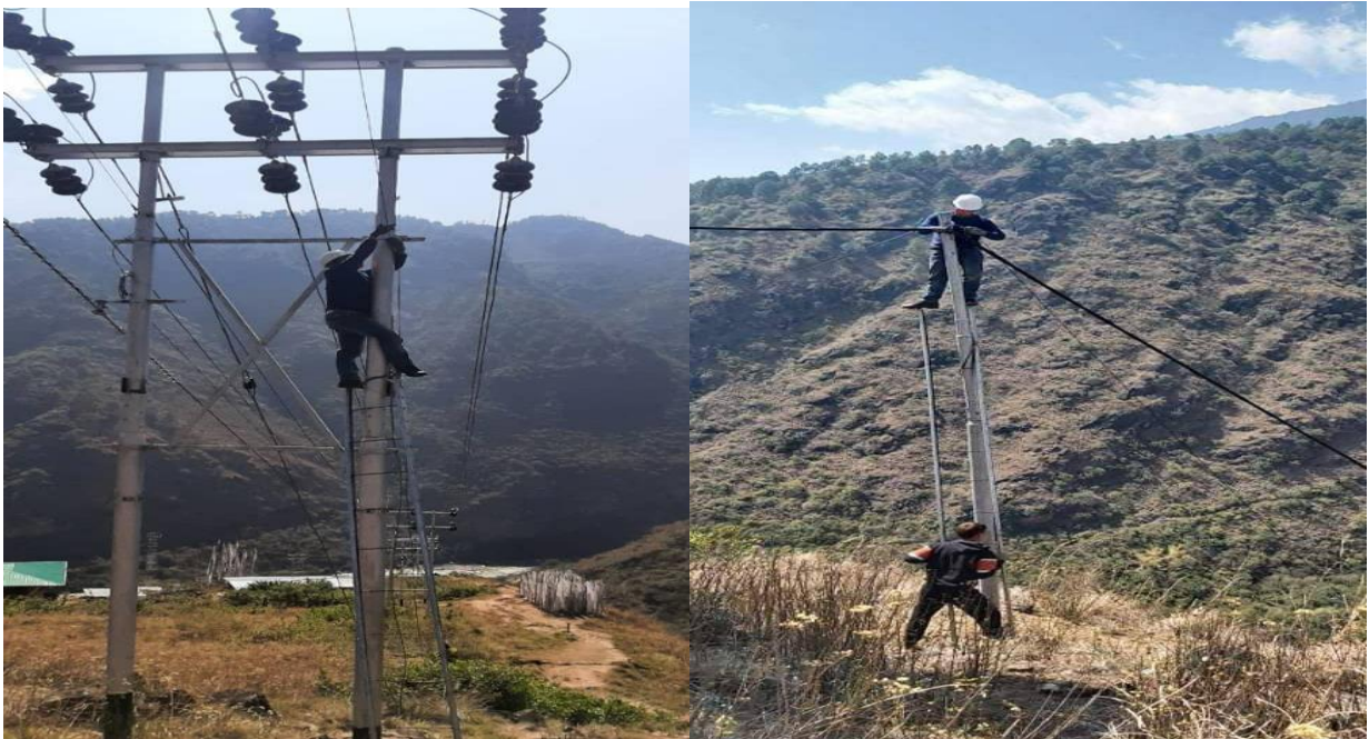
Figure 8. LCOs of Tashi Yangtse Doksum maintaining the cable line (26, February, 2022)
