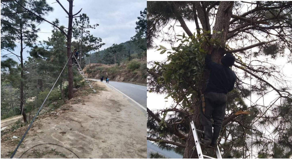
Figure 7. LCOs of Punakha rectifying the cable line after the snowfall (January,2022)
