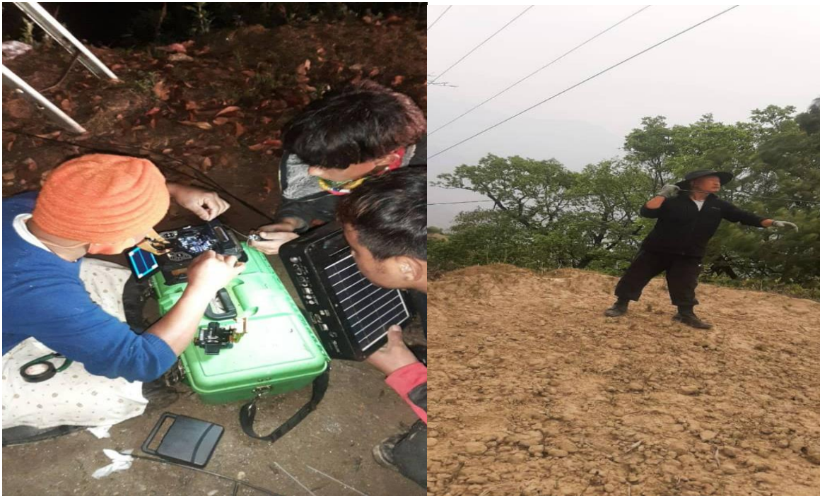
Figure 10. LCOs doing the cable maintenance (23 March, 2022)
