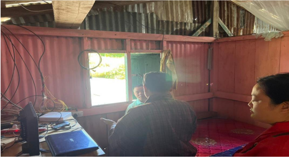
Figure 11. Control room and meeting with NL Cable Service
