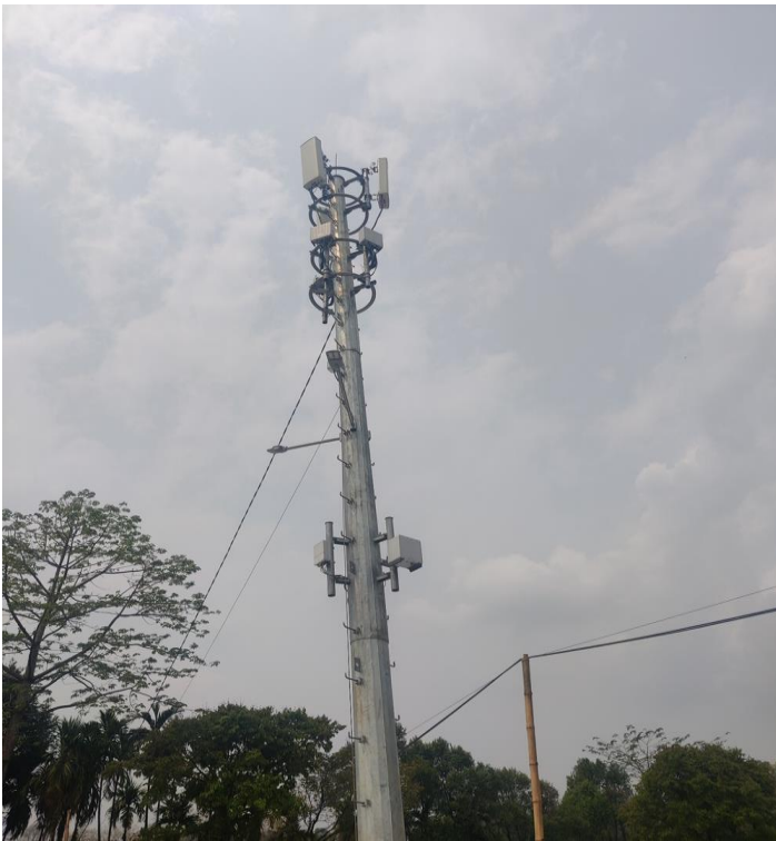
Figure 49: Samtse Check post D-Site (BTL)
