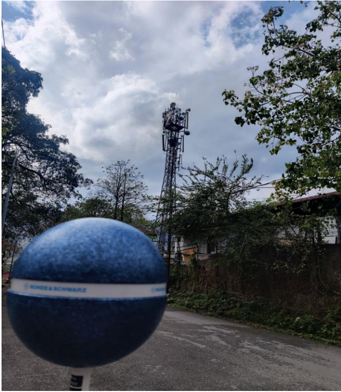
Figure 43: Phuntsholing TX (TICL)
