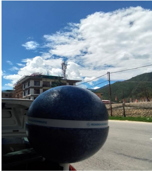
Figure 54: Upper Taba (TICL) 3 Legged Tower.
