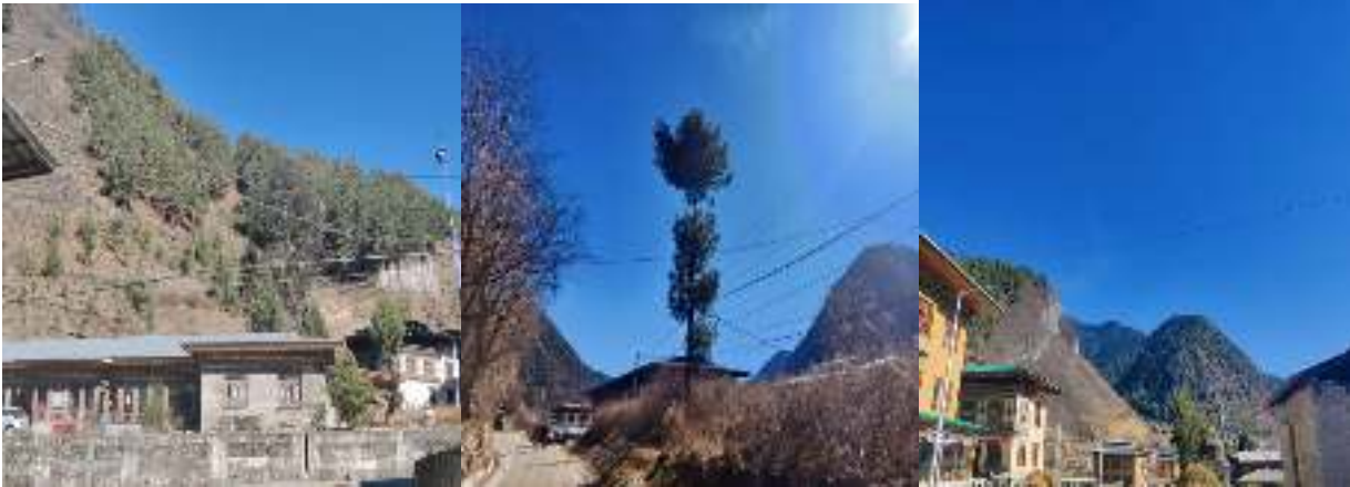
Figure 21: Non usage of poles for cable road cross over by Leki cable and hanging cables at road cross over at Haa Town
