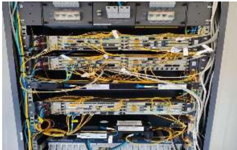
Figure 14: DWDM of TICL for international bandwidth connection with TATA at Pasakha BTS site
