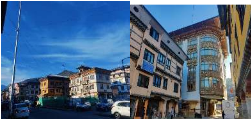
Figure 29 : Low hanging cable of BTL with cables criss crossing each other at Paro town
