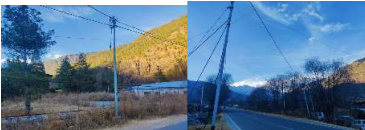
Figure 34: Low hanging cables ( at ground level near Zhiwa Ling hotel ) near Satsam chorten, hanging cables near Kichu lhakhang of Sigma cable
