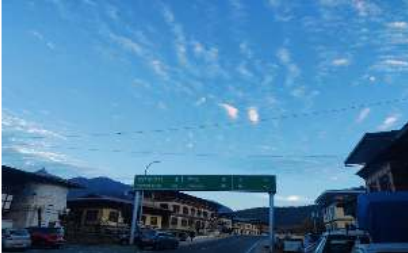
Figure 37 : Multiple rooftop to rooftop road cross over though there are available poles for common cable road cross over at Bondey town for Both TD and Sigma cable
