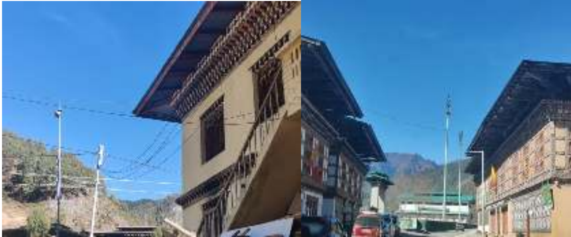
Figure 24: Multiple rooftop to rooftop cable road crossover by Leki cable at certain places of Haa Town.
