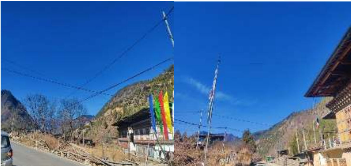
Figure 22: Non usage of poles for cable road cross over by Leki cable and hanging cables at road cross over at left - near the bridge below Lhakhang Karpo and right- Katsho area.
