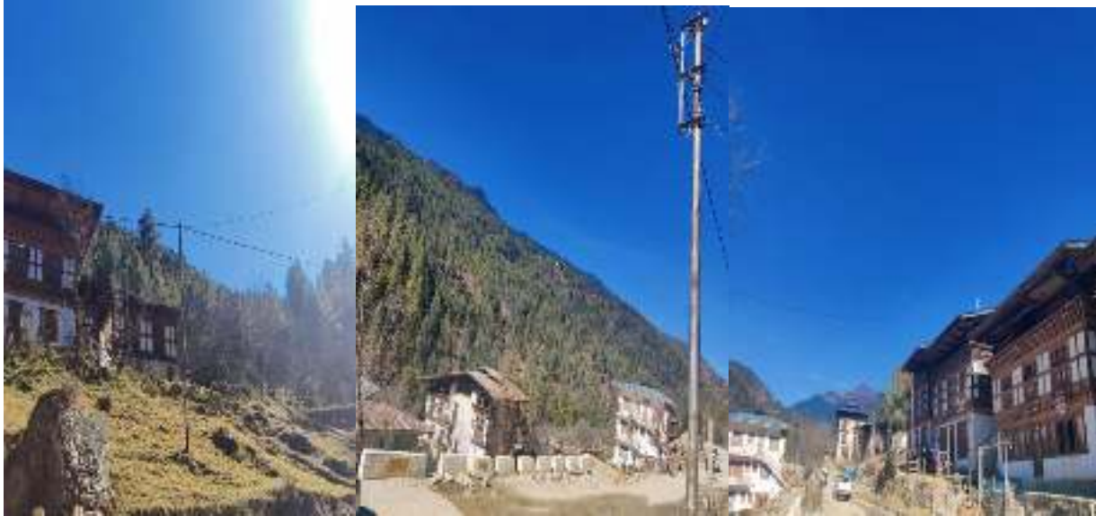
Figure 25 : Non usage of poles for common cable road crossover by Leki cable at Gjenkana area, Samar Gewog, Haa
