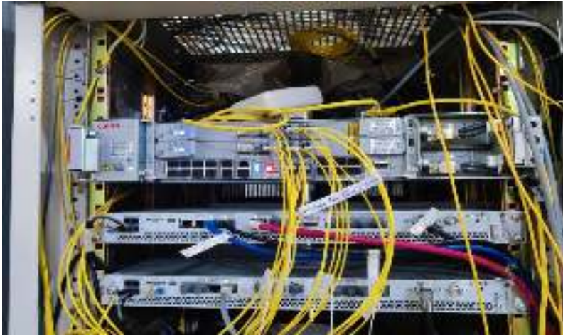
Figure 13: DWDM of BTL for international bandwidth connection with TATA at Pasakha BTS site
