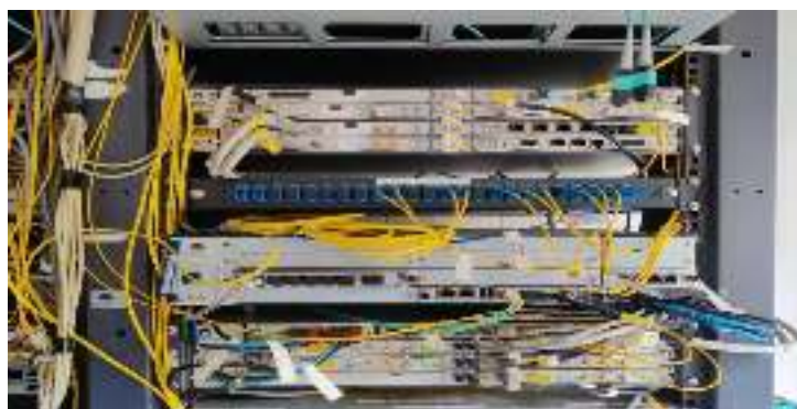
Figure 10: The DWDM equipment of TICL at Phuentsholing main site for International bandwidth connection with Airtel
