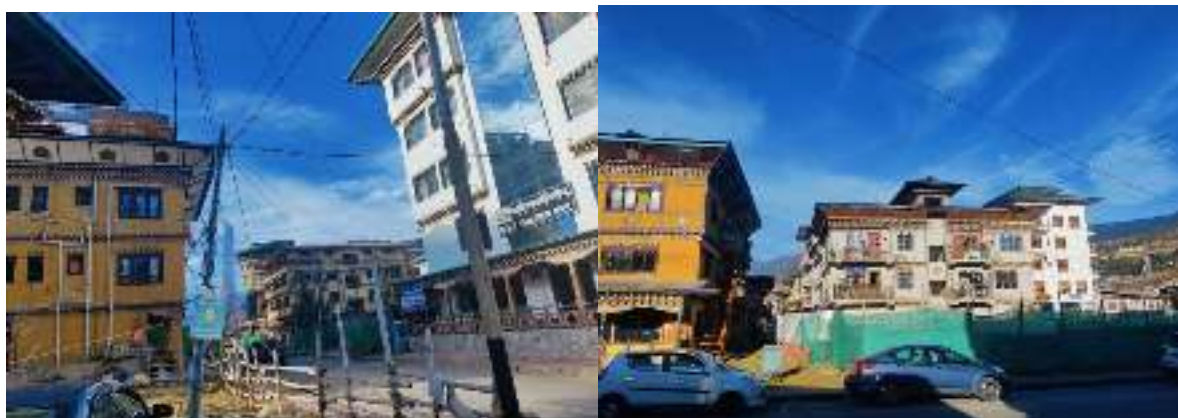
Figure 30: Low hanging cable at BTL's pole sharing site
