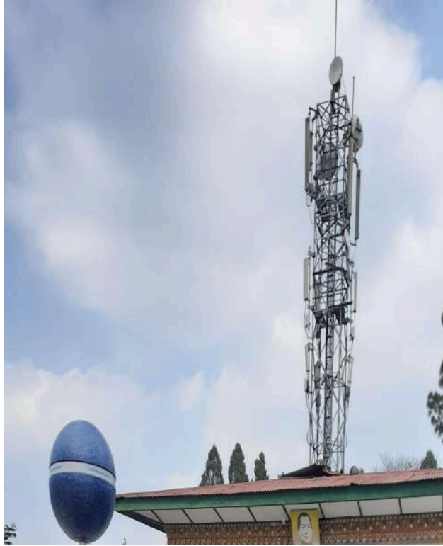
Figure 21: BTL main Exchange, Damphu
