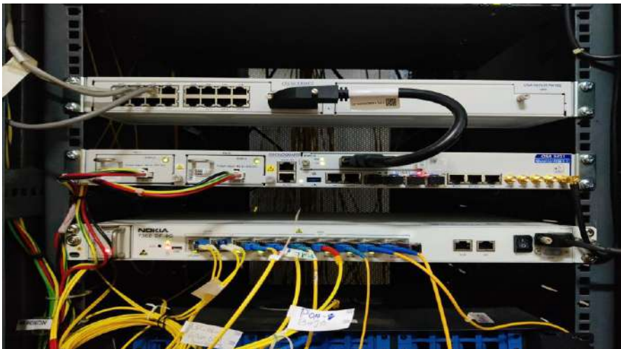
Figure 16: FTTH(GPON- Nokia) installed at Wangdue BTL Office
