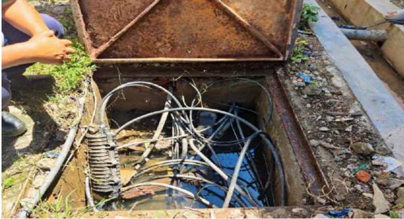
Figure 17: Underground duct system for communication services at Bajo Town
