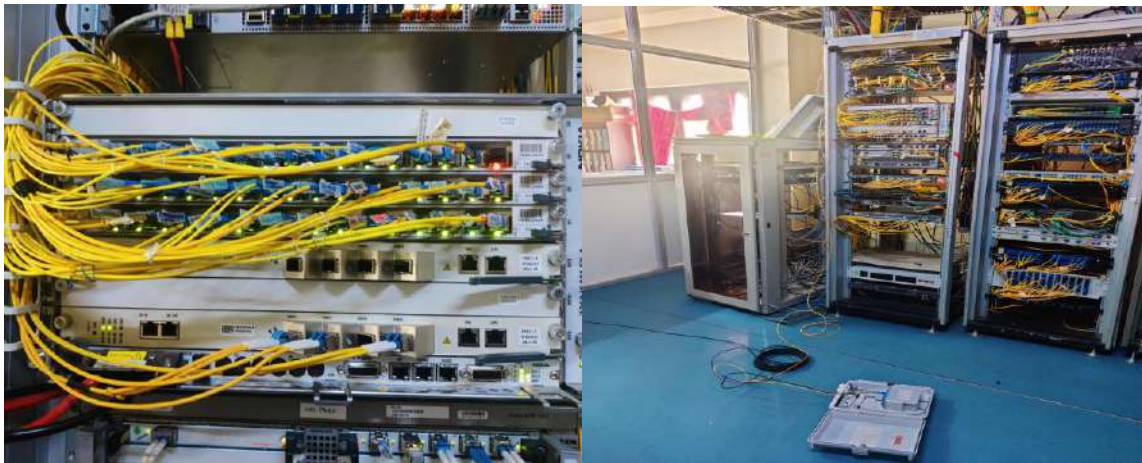
Figure 10: FTTH(GPON) equipment installed at Paro BTL Office
