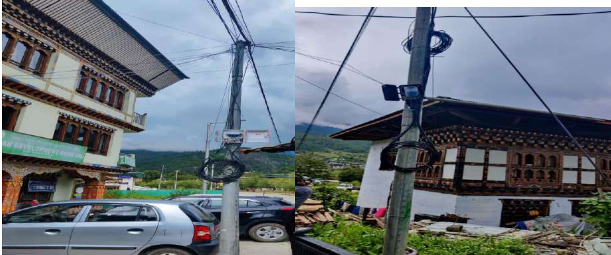
Figure 2: FTTH splitters at various locations at Haa Town for fiber network distribution.
