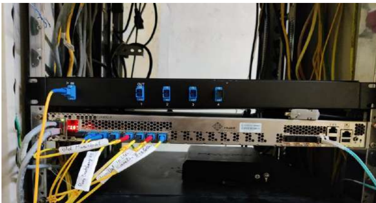
Figure 20: FTTH equipment (Tejas) installed at Khuruthang BTS site
