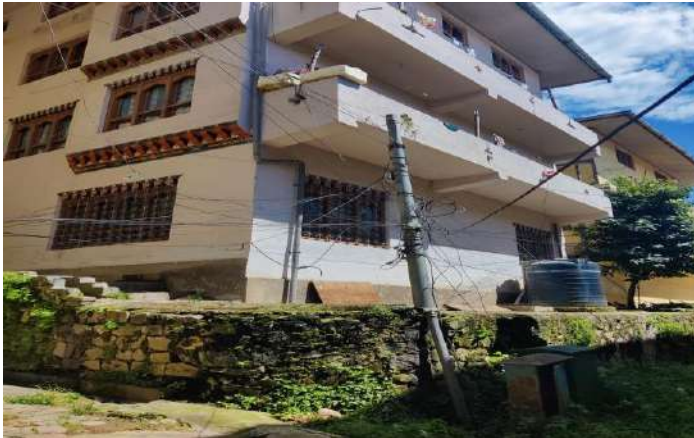
Figure 18: Low Hanging cables around the pole sharing sites.
