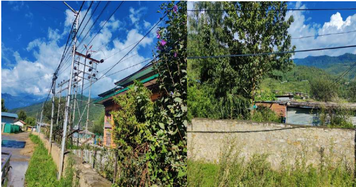
Figure 14: Low hanging stray cables of TD Metho(left) and Sigma cable service(right) on the roads towards Dhopsahri Gewog center.
