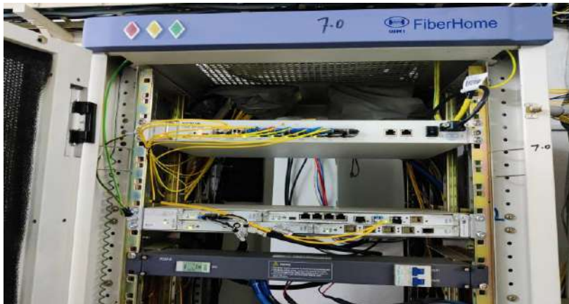
Figure 1: Nokia GPON equipment installed at Haa BTL office as part of FTTH part network
