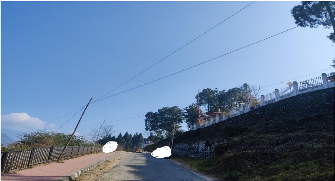
Figure 3 : Non usage of Poles for cable road crossover despite poles available for sharing by BTL and T&T cable near Dagana Dzong area
