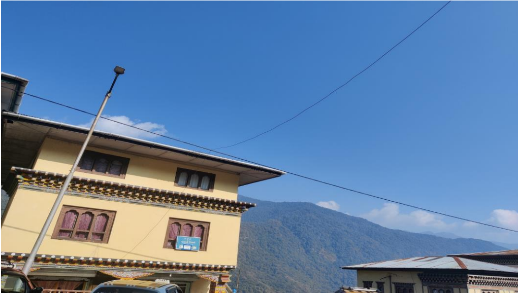
Figure 2: Low hanging cross over cable of T & T cable in Dagana town
