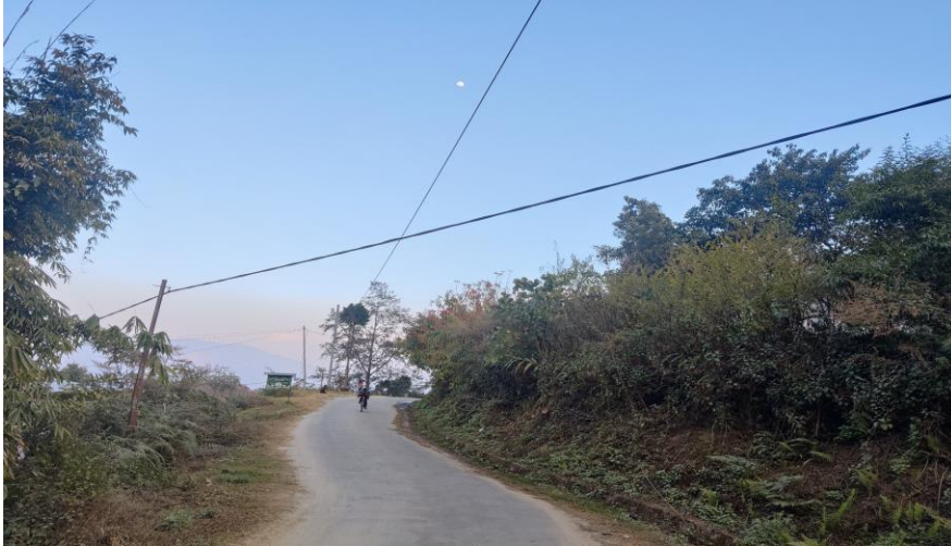
Figure 5: Low cable road cross over of BTL in Dagapela Town
