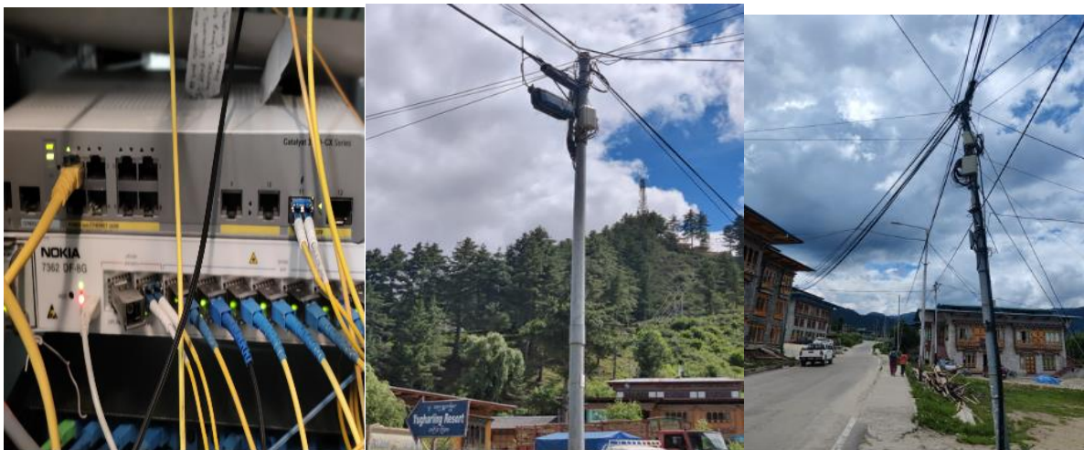
Figure 9: Nokia GPON OLT with splitters (FTTH network) in Jakar town and its peripheral areas
