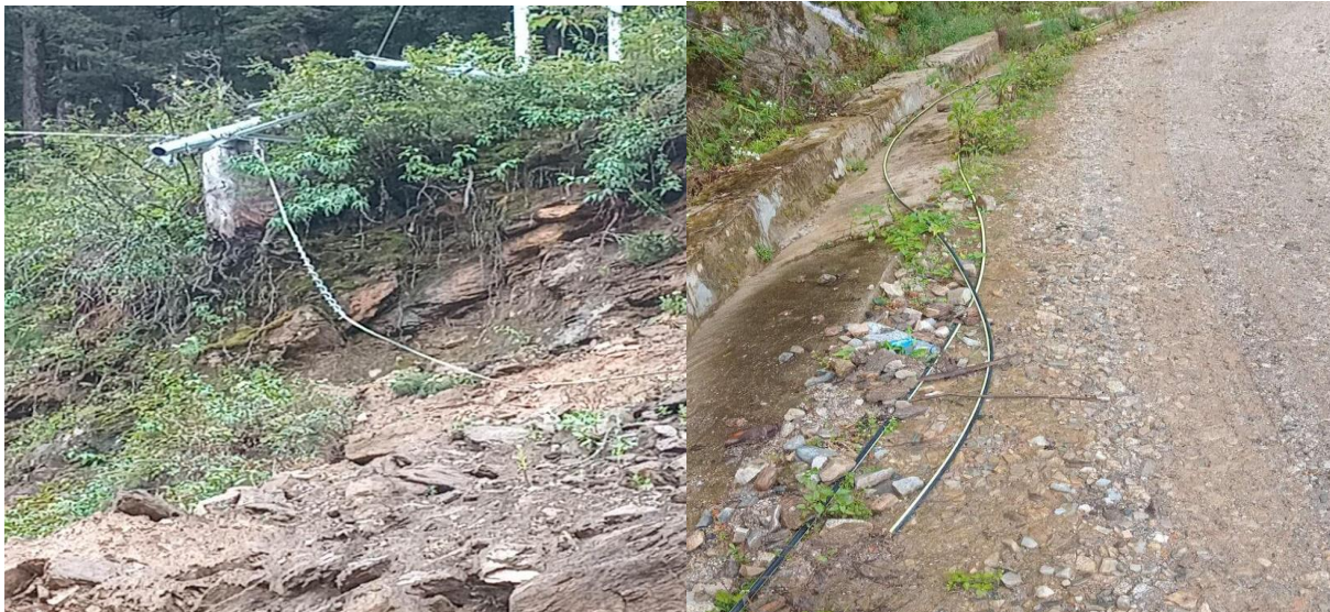
Figure 2 : ADSS fiber damaged enroute to Naro gewog Center
